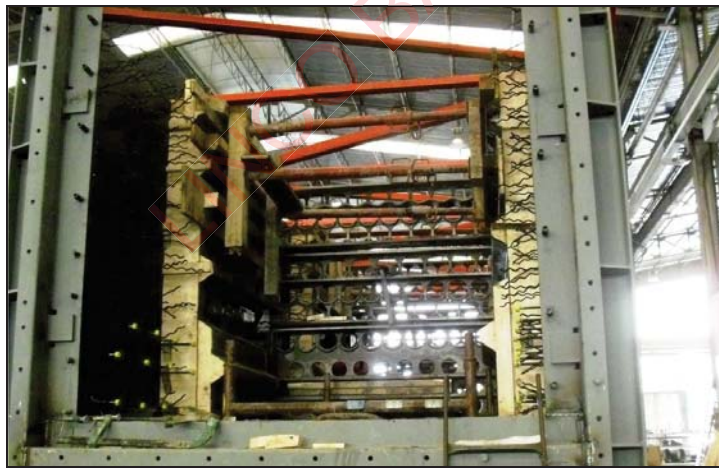
Convection corbels shuttering of a petrochem heater
