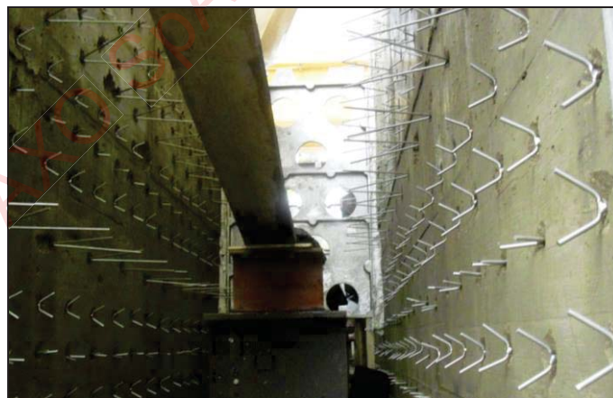
Metallic anchors welded on a convection wall
