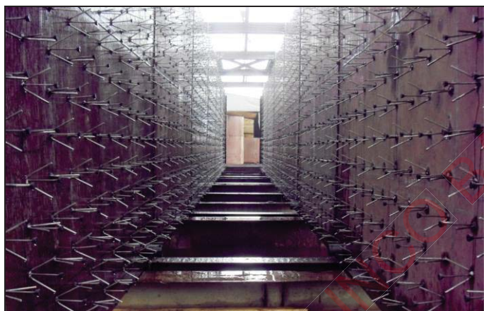
Metallic anchors welded on a convection wall
