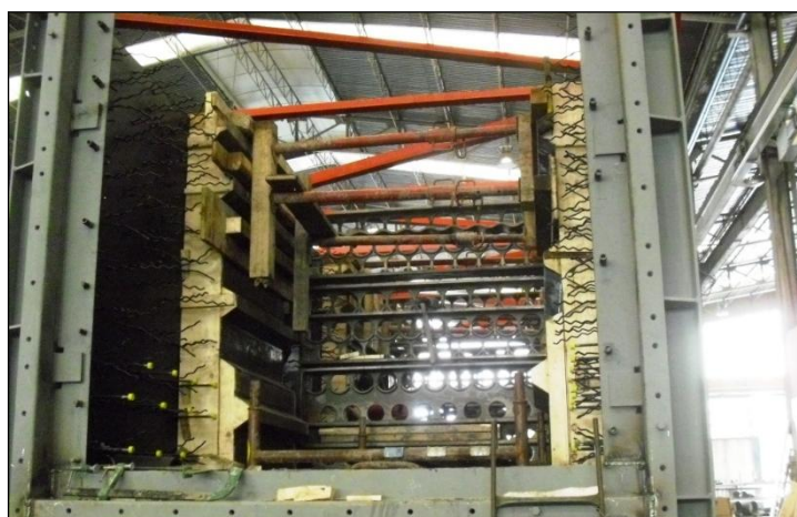
Convection corbels shuttering of a petrochemical heater
