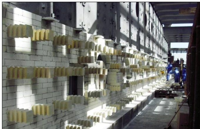
Ceramic anchors on a side wall of a reheating furnace
